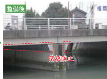
橋梁の耐震補強
