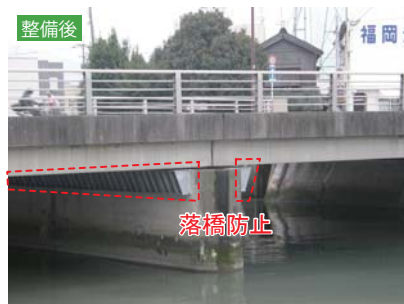
橋梁の耐震補強
