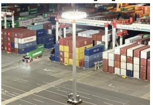
Conversion to LED lighting has reduced power consumption compared to conventional sodium lamps.
