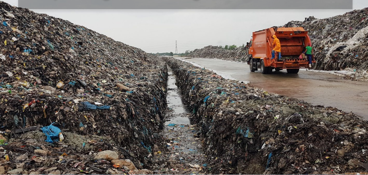
Improving the drainages around the cell
