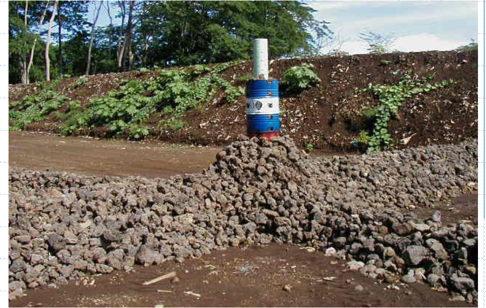
Perforated Gas Venting Pipe
