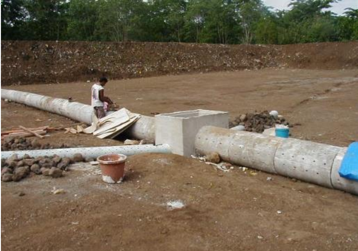
Perforated Leachate Collection Pipe on the slightly inclined base
