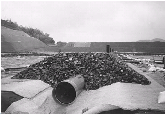
Main collection pipe (under construction)
