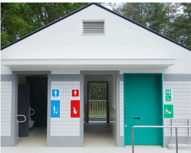
Appropriately-sized signs have been installed, and the use of distinctive colors on the signs makes them easily recognizable as toilets from a distance.
