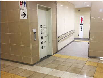
Eliminating steps at toilet entrances (ramp conversion)
