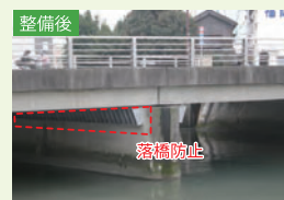
橋梁の耐震補強
