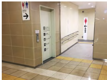
Eliminating steps at toilet entrances (ramp conversion)
