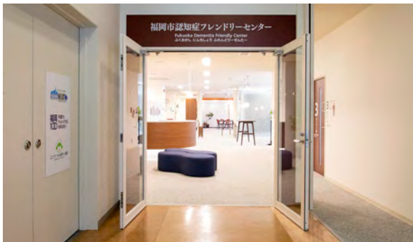
Signs in colors that contrast with the surroundings are installed so that they are easily recognizable.
