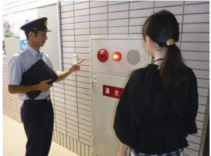
▲立入検査 On-site inspection
