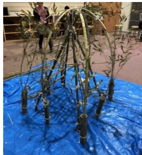
Fig. 3 An example of a bamboo fish reef made in a citizen participation course
