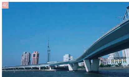
Fukuoka Urban Expressway Route 1, Bridge over the Muromi-gawa Riv.
