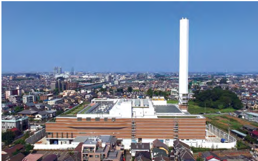
Nerima Waste incineration plant (Tokyo, JAPAN)
