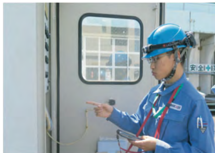
Maintenance and inspection
