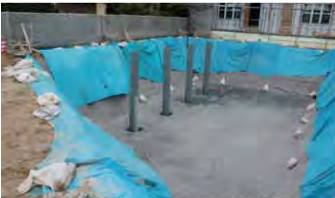
④ Filling with crushed stones
