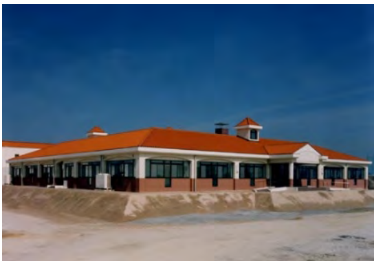
<Yukuhashi-Shi, Fukuoka, Japan Sewage treatment center>
