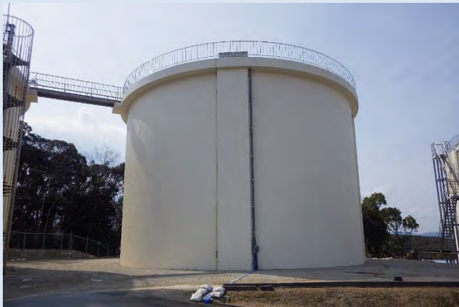
PC storage tank for drinking water
