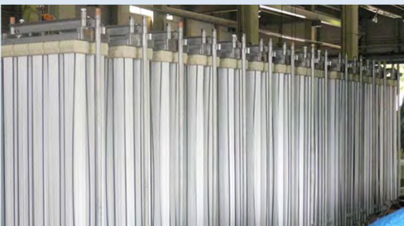
■ Submerged PTFE MF membrane
