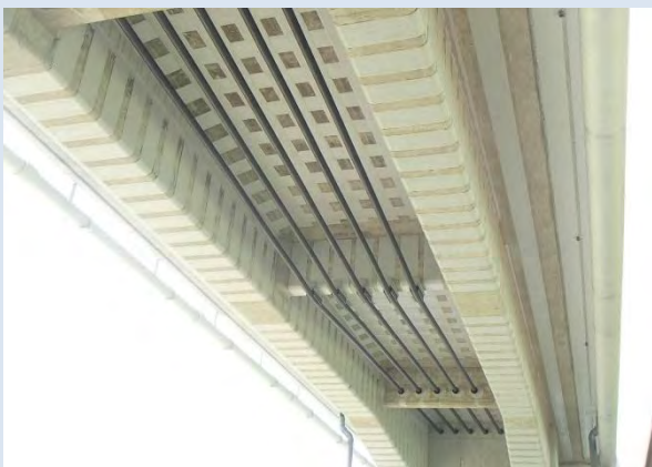
<Reinforcement of external cables> <Reinforcement of carbon fiber sheets>
