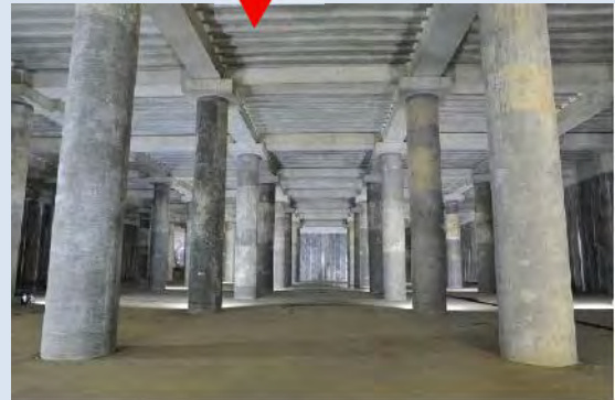
Retention Basin (for when heavy rain falls)
