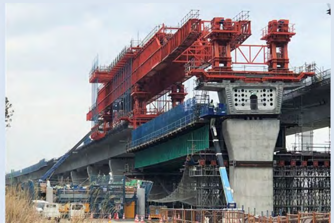
Span-by-Span Precast Segment Method
