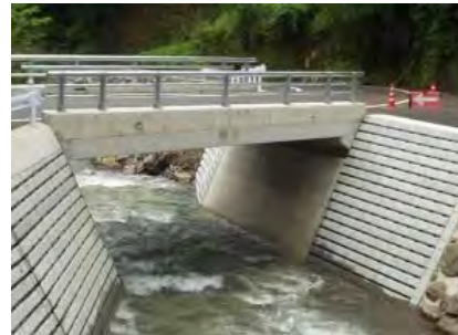
Place : Kumamoto prefecture, Taraki town Construction year : April, 2013 FA BOX
