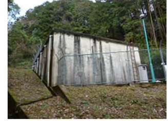
Seismic diagnostic for Mizukigaoka Distributing Reservoir
