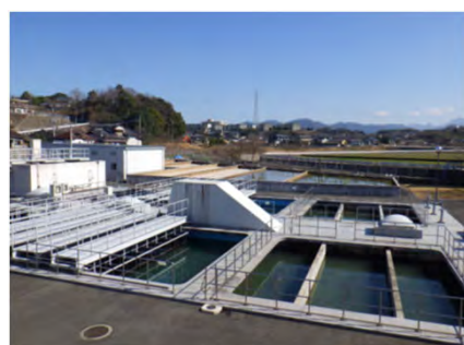
Industrial water settling tank
