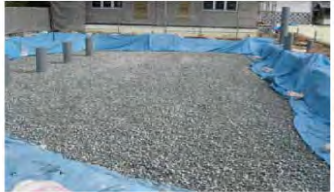
⑥ Surface compaction
