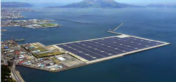
< Nanatsu Island Mega Solar Power Station > (Max output of 70MW)
