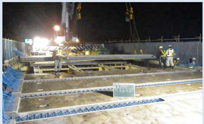
<PC slab Replacement Method>
