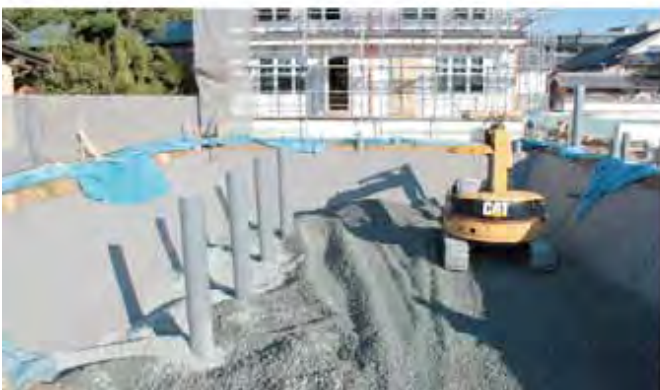
④ Filling with crushed stones
