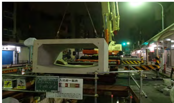
<Tokyo, Sewage Box culvert pipe>
