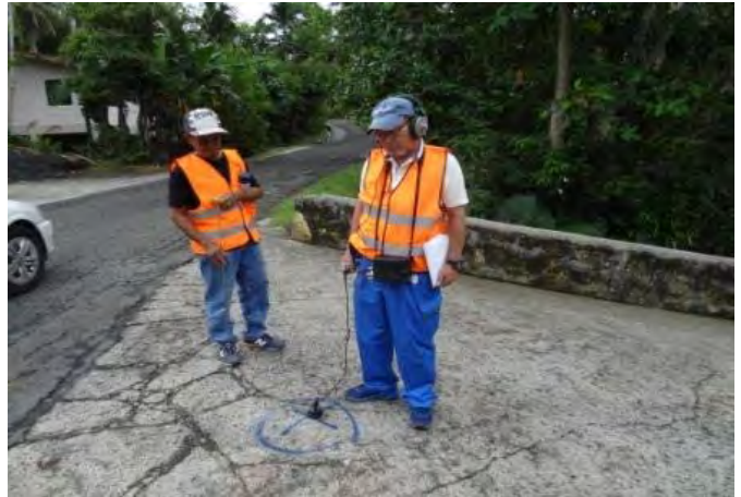
(LEAKAGE SURVEY AT PALAU)
