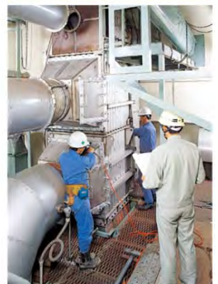
Incinerators heat exchanger replacement (high efficiency and energy saving)
