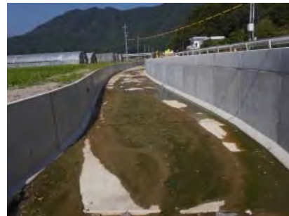
Place : Oita prefecture, Saiki City Construction year : March, 2015 YT Ditch H-1500
