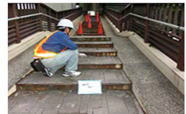
Investigation for maintenance of installed stairs of Najima Benten Bridge
