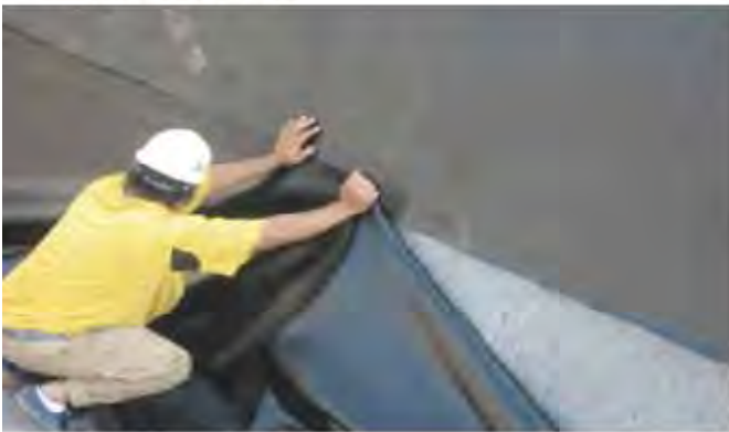
③ Installation of the intake pipes
