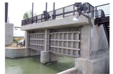
Inverted design of agricultural water channel
