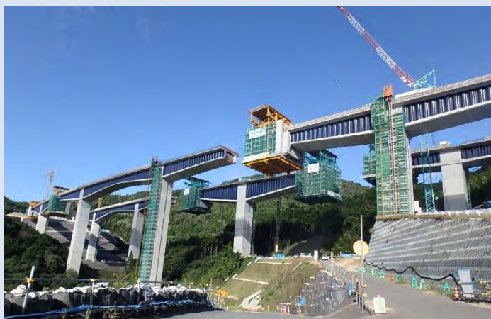
<Cantilever Method> Corrugated Steel Sheet Web
