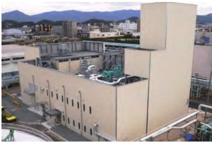
Sewage sludge solid-fuel conversion facility
