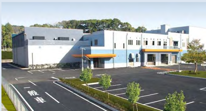
< Sludge Recycle Treatment Complete view >
