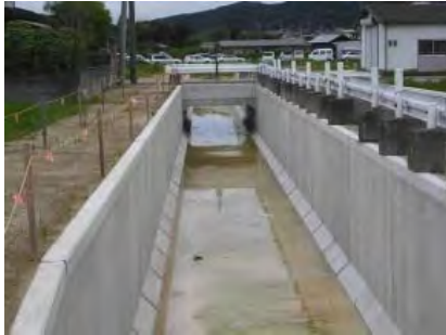
Place : Oita prefecture, Oita City Construction year : April, 2015 Box Culvert (3500×1500)
