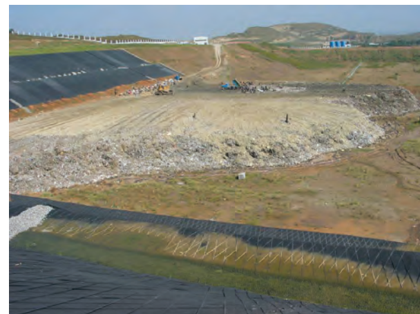
Filling in landfill (2003)
