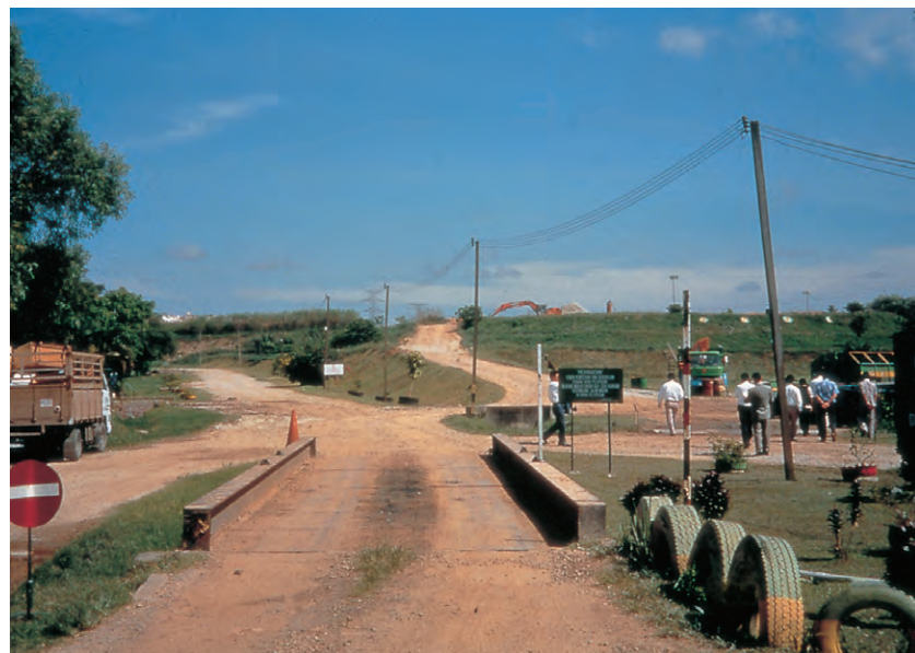
The Ampang Jajar Landfill after improvement (1996)
