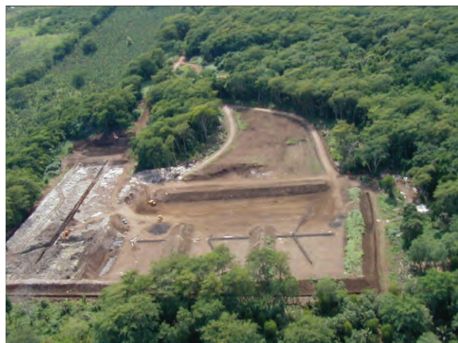
Ongoing improvement of landfill through the Fukuoka Method (2003)
