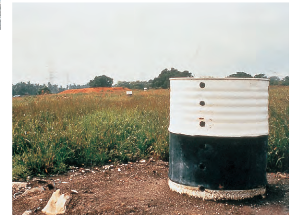
Vegetation recovery after the installation of the gas ventilation system
