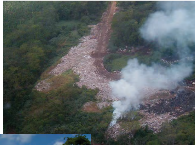
Conditions of landfill before improvement (2001)
