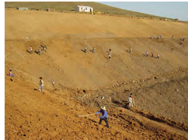
Forming slope before impermeable liner installation (2002)
