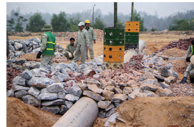
Installing gas collection pipe and ventilation system built from waste steel drums (Nam Son Landfill, Hanoi City, Vietnam) (2005)
