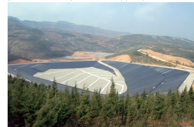
Completed landfill site (2007)
