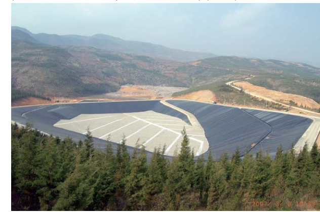
Completed landfill site (2007)
