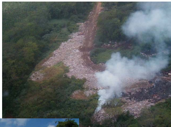
Conditions of landfill before improvement (2001)
