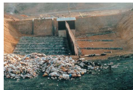
Field experiment at Hisayama Landfill (1974) Left: Aerobic landfill, Right: Semi-aerobic landfill
