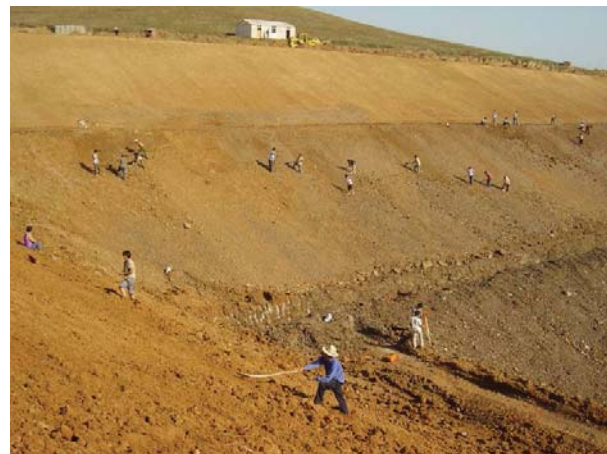
Forming slope before impermeable liner installation (2002)
