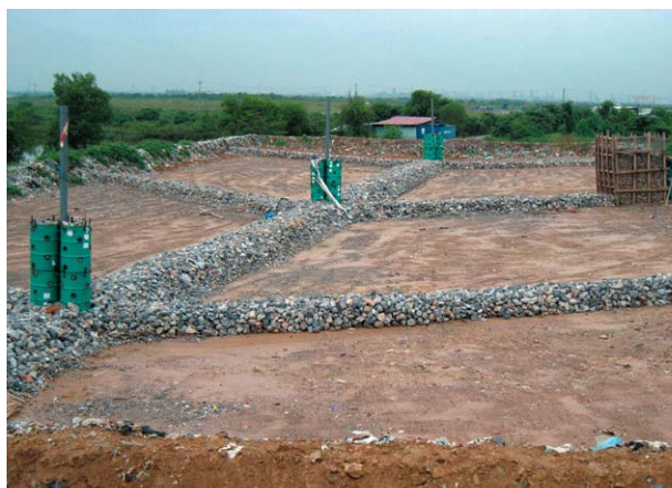
Ongoing improvement of landfill through the Fukuoka Method in Dinhvu, Hai Phong City (2011)
