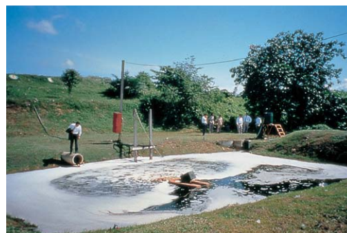
Aeration in the retention pond (1996)
