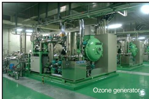
This water treatment plant treats 122,000 m<sup>3</sup> of water a day through coagulation, sedimentation, rapid filtration and other advanced water treatment techniques (such as ozone treatment and granular activated carbon adsorption treatment).
