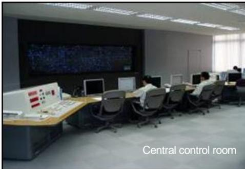
The center monitors the ever-changing water consumption level in the city **24 hours a day**, and adjusts the water pressure by remotely-controlling an electric valve.
