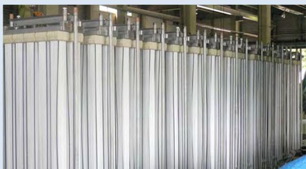
■ Submerged PTFE MF membrane
